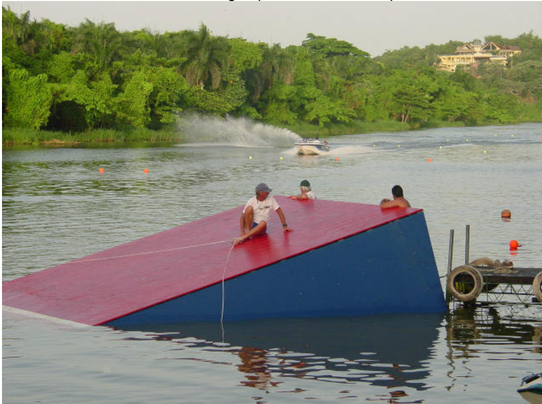
The "Slew Crew" getting ready to install the ramp.
